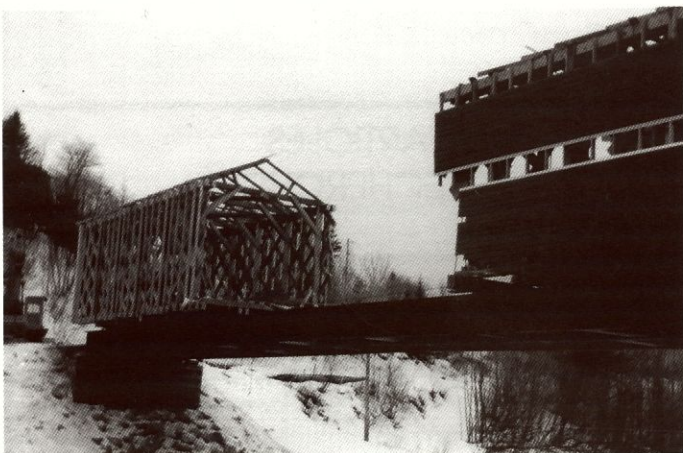
Le pont Louis-Gravel (61-62-01) Photo: André Cloutier ©
