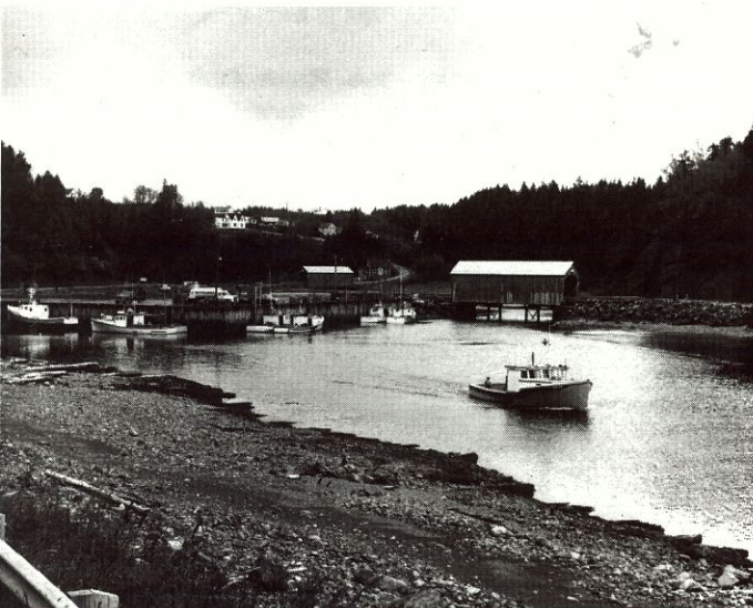
Saint Martins; les ponts Vaughan Creek (55-11-05) et Hardscrabble Hill (55-11-06). Photo: Joseph D. Cornwill ©
