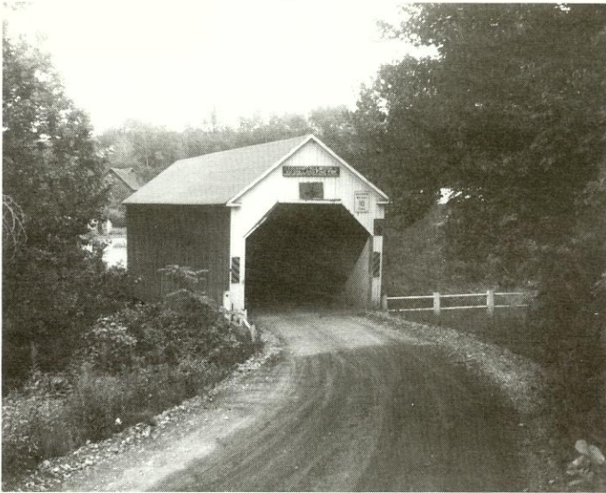
Le pont Lockhart Mill (55-02-09) Photo: Joseph D. Conwill ©
