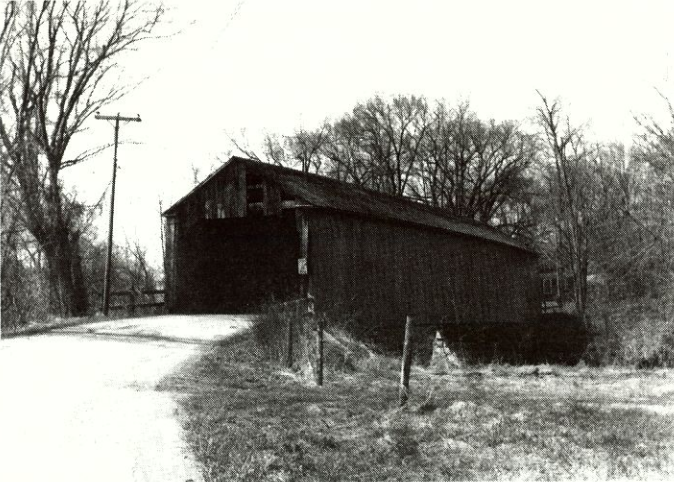
Pont Sanderson (45-11-02) PHOTO: Joseph D. Conwill, 1974 ©
